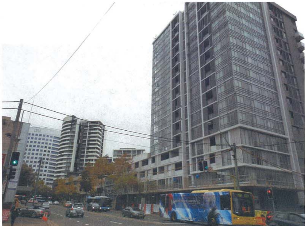
Figure 7: Photo of the adjacent 16 storey mixed use development to the north with a 4 storey podium. The 20 storey Abode and 20 storey IBM building are also shown (left) (Source: CPSD).
