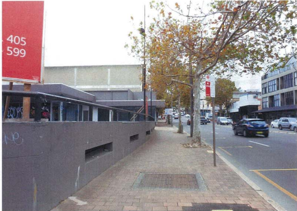
Figure 4: Photo of the primary street frontage of the existing site as viewed along the Pacific Highway looking south-east (Source: CPSD).
